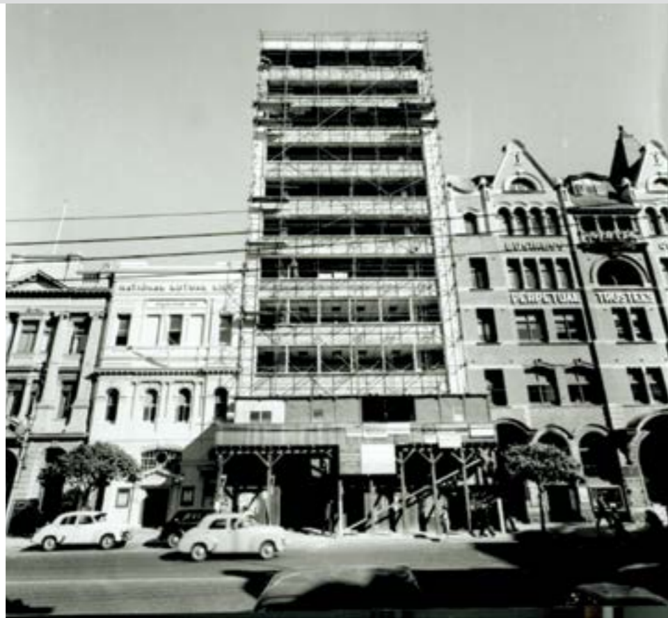
The National Mutual Building under construction in the mid-1950s.
