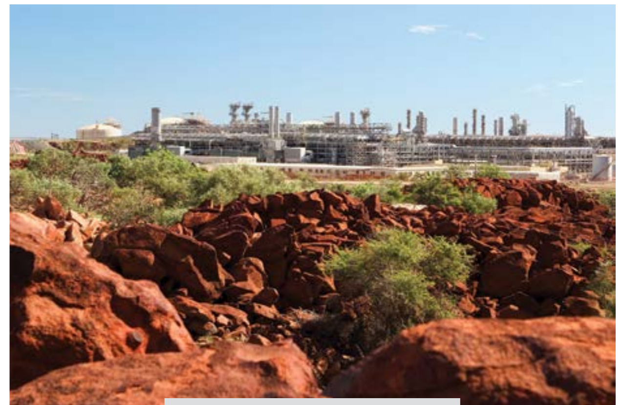
Woodside Karratha Onshore Gas Plant
