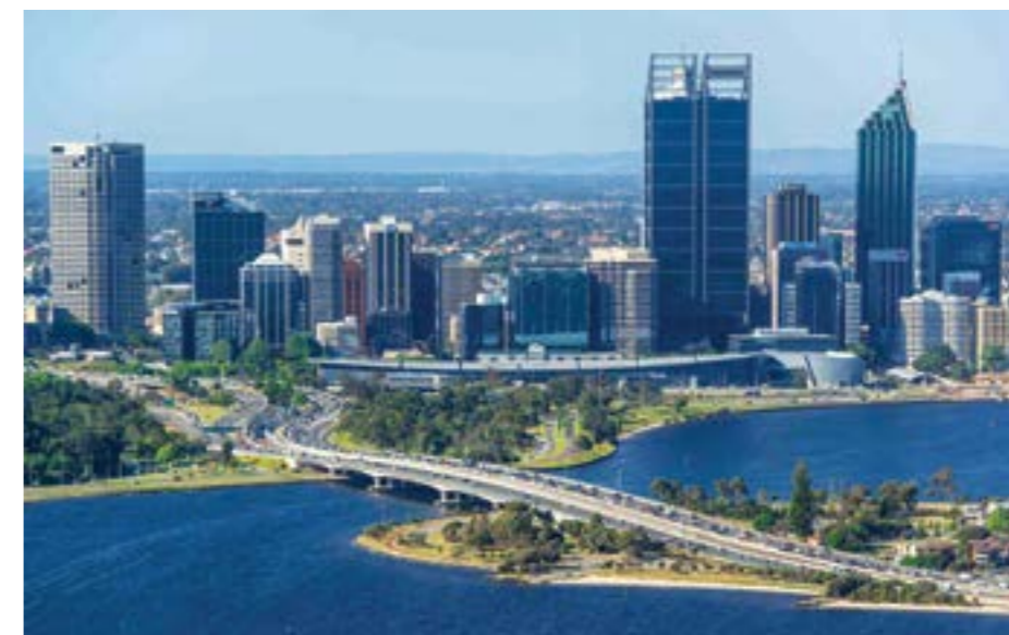
Position of the Narrows Bridge today, with the new Clough building centre right
