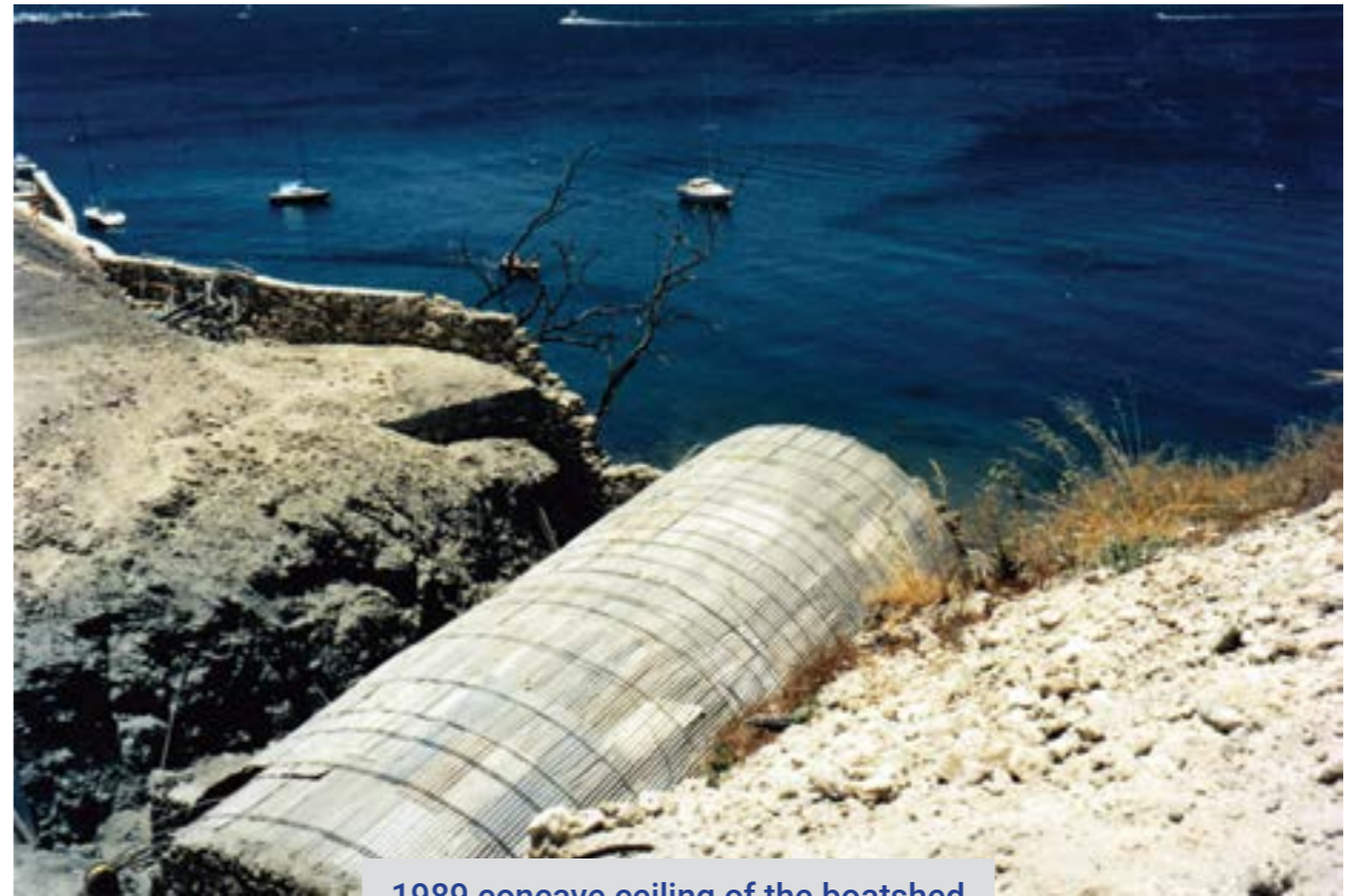
1989 concave ceiling of the boatshed
